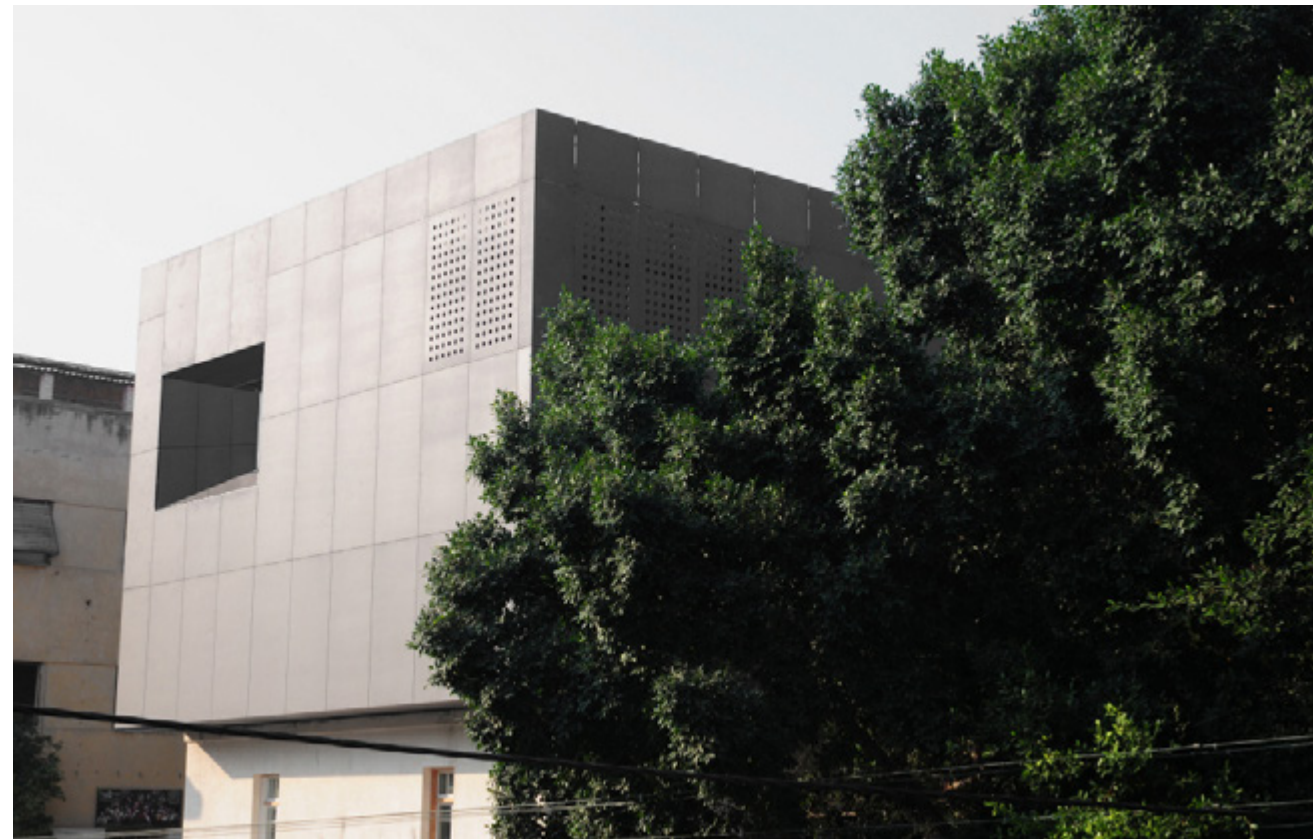
North East wing facade
